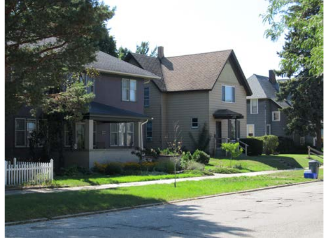
Traditional single family housing units in Ludington.
